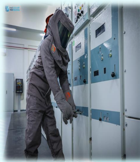
Added medium voltage network lengths 124.3 KM
